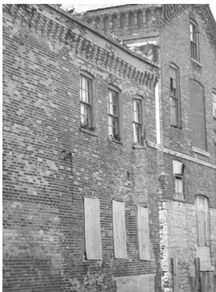
Figure 4.9. Detail of the north facades of the 1860s brick buildings. Notice the bricks curving inward between the windows. See also the first floor window damage. Image by author.
