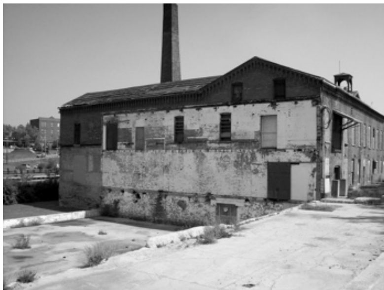
Figure 4.10. West façade of 1860s brick building. The Canal is in the background. Note areas of brick failure, particularly at the ground floor level. Image by author.
