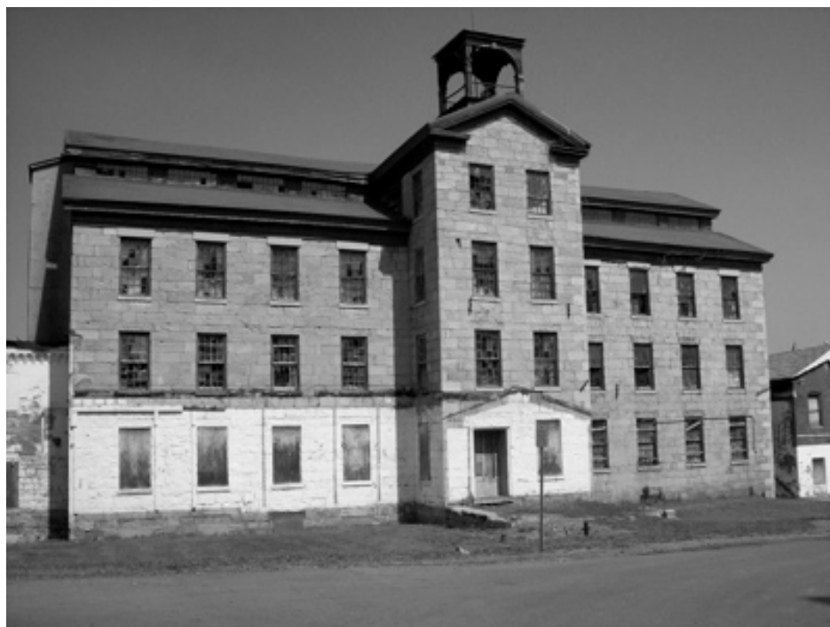
Figure 4.2. 1844 Stone mill building, south façade. Note the window damage and ghosting at the ground floor level. Image by author.
