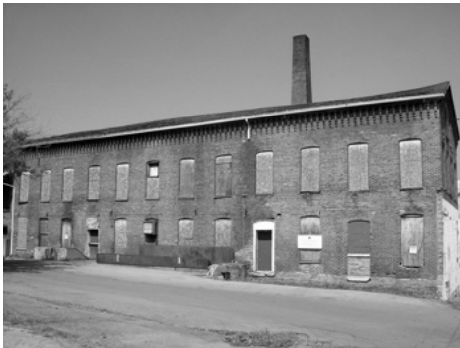
Figure 4.8. Detail of south façade of one of the brick buildings. Note the smokestack and the brick corbelling under the eaves. Image by author.
