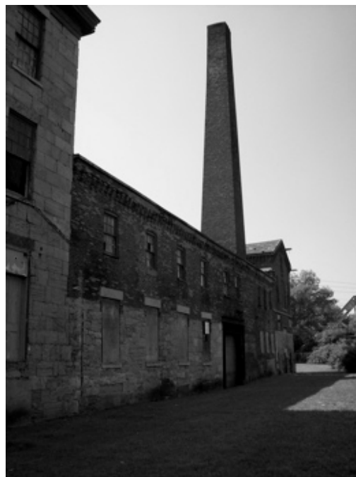
Figure 2.10. Modern day photograph of the 1860s brick additions. The two-and-a-half story structure at the west continues back farther than the south façade of the two-story brick structure, forming an L-shape plan. Image by author.
