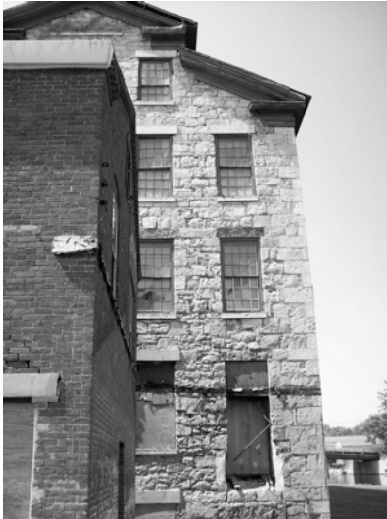
Figure 4.5. Stone building, east façade. Note the twelve-over-twelve windows, stone sills and lintels, and the quoins at the corner. Ghosting and window damage also noticeable. Image by author.
