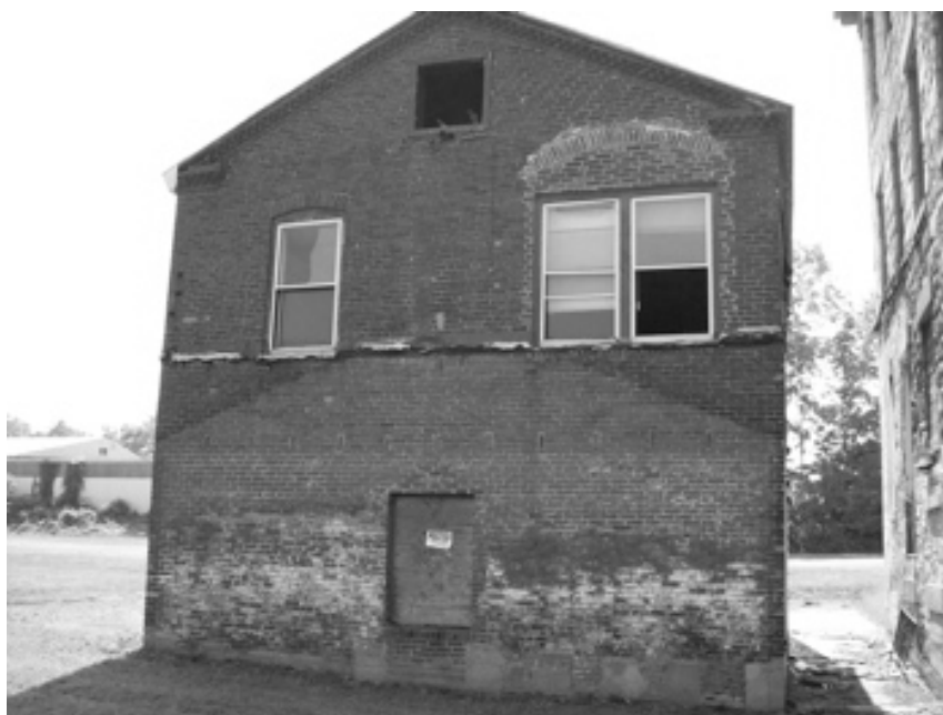
Figure 4.13. North façade of brick building. Note the efflorescence near the base of the building and surrounding the second floor window. Image by author.
