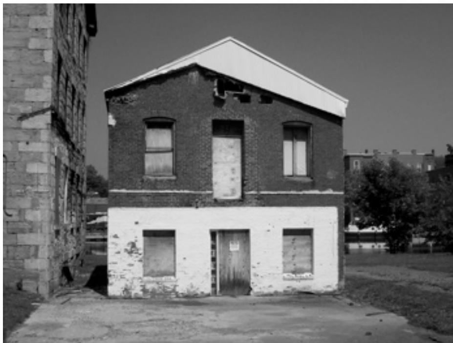
Figure 4.12. South façade of the brick building to the east of the stone building. Note the windows, brick failure at the roofline, and growth at the ground line. Image by author.
